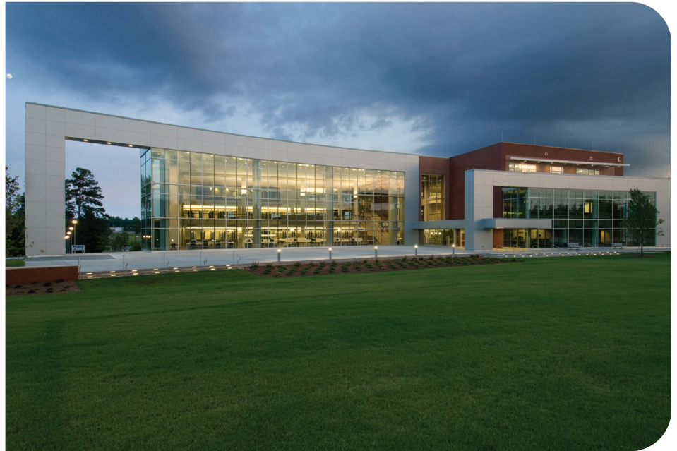
The GGC Library, which was designed by LEO A DALY, Atlanta, features Solarban ® 70 Starphire ® glass by Vitro Architectural Glass (formerly PPG glass) and a curtainwall system by Kawneer. Both are Cradle to Cradle Certified ™ .
