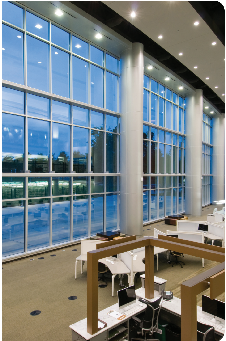
The large atrium at the GGC Library provides 75 percent of the interior space with natural daylight. With VLT of 64 percent and SHGC of 0.27, Solarban® 70 Starphire® glass achieves a light to solar gain (LSG) ratio of 2.37.
